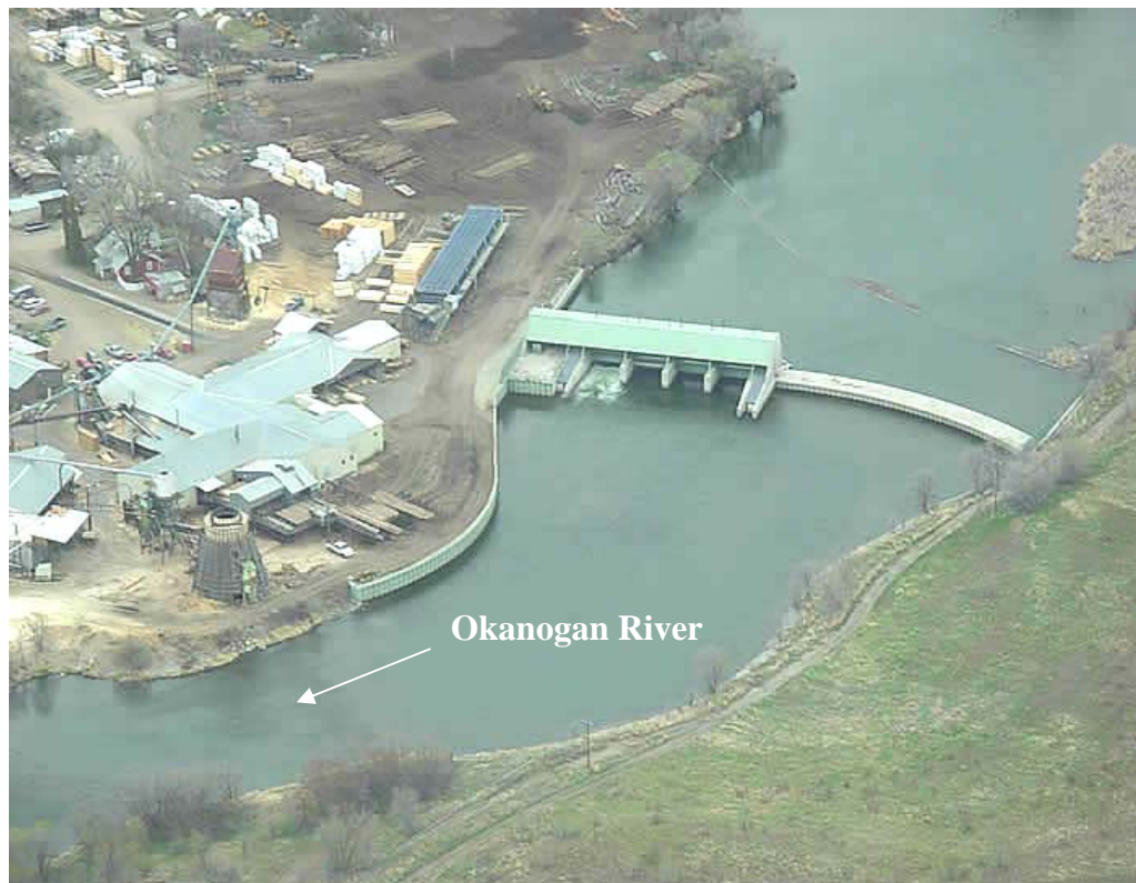
Figure 2.3 Aerial view of Zosel Dam indicating the control structure and overflow weir.
