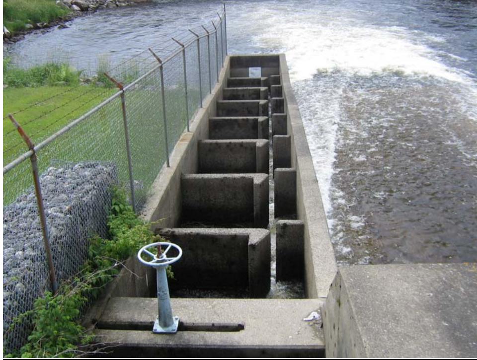
Vanceboro Dam, June 2011, flow through gate next to fishway
