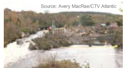
November 2023, Milltown Dam structures
