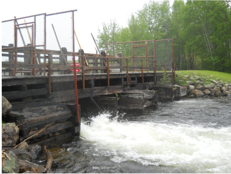
Forest City Dam (6-4-2014), View of dam from downstream.
