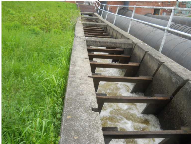
Grand Falls Dam (6-4-2014), View of Denil fishway alongside powerhouse.
