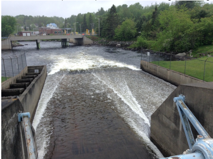
Vanceboro Dam (6-4-2014). View of flow through Tainter gates.
