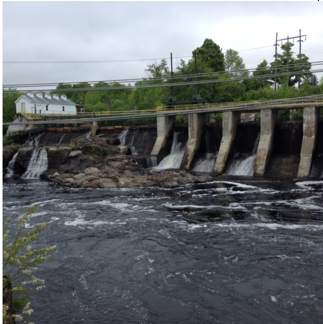
Milltown Dam (6-4-2014), View of spillway and powerhouse.
