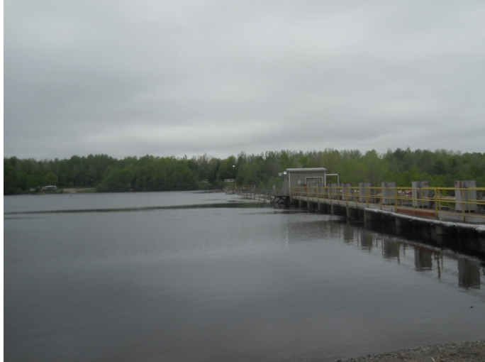
Grand Falls Dam (6-4-2014), Upstream side of spillway from US side.
