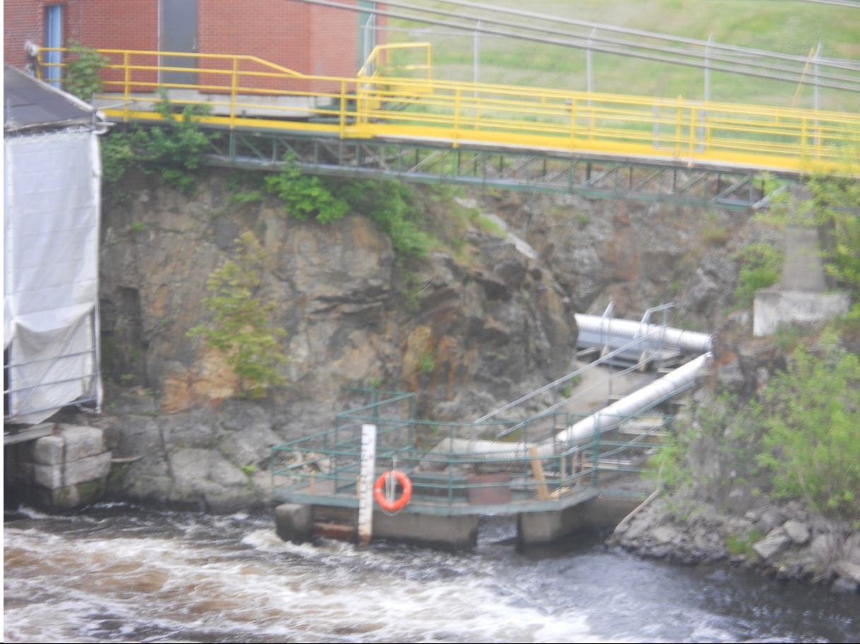
Milltown Dam (6-4-2014), View of fishway.
