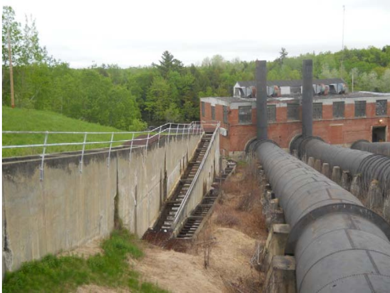
Grand Falls Dam (6-4-2014), View of Denil fishway above the powerhouse.
