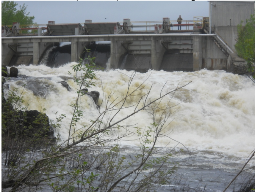
Grand Falls Dam (6-4-2014), View of Tainter gates from downstream.
