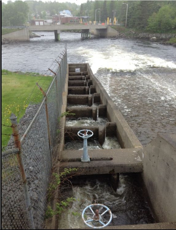
Vanceboro Dam (6-4-2014), View of fishway.
