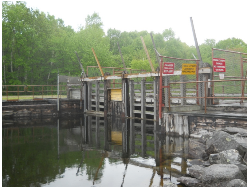
Forest City Dam (6-4-2014), View of gates from upstream.
