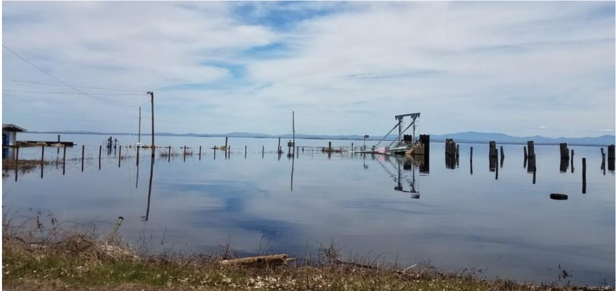
Port Kent ferry dock on New York side of Lake Champlain during minor flooding in 2019. Photo Credit: Eric Day
