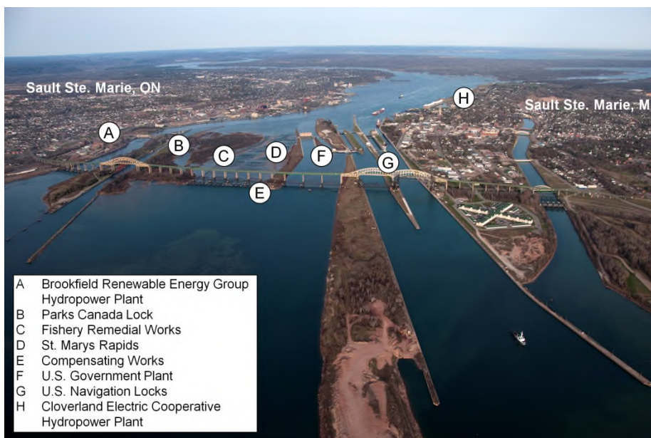
Structures at the head of the St. Marys River that control the outflow from Lake Superior.
