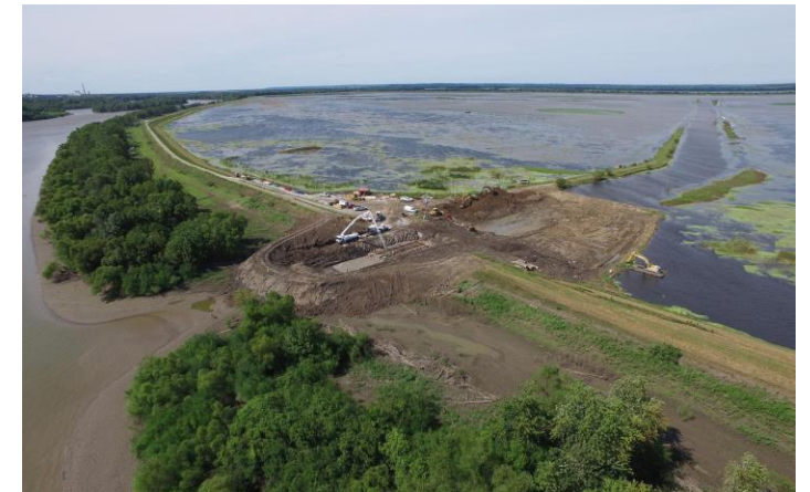
Berm removal on Otter Creek 2019-02-15
