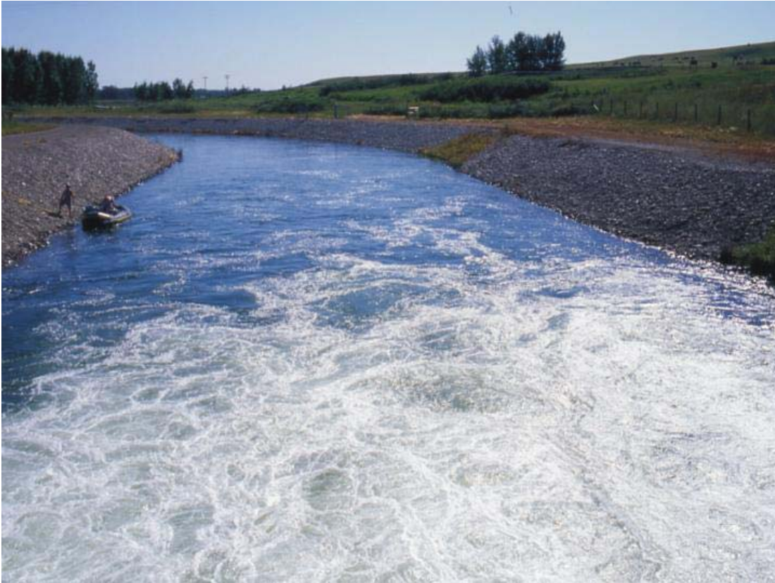
Carseland Bow Headworks Canal
