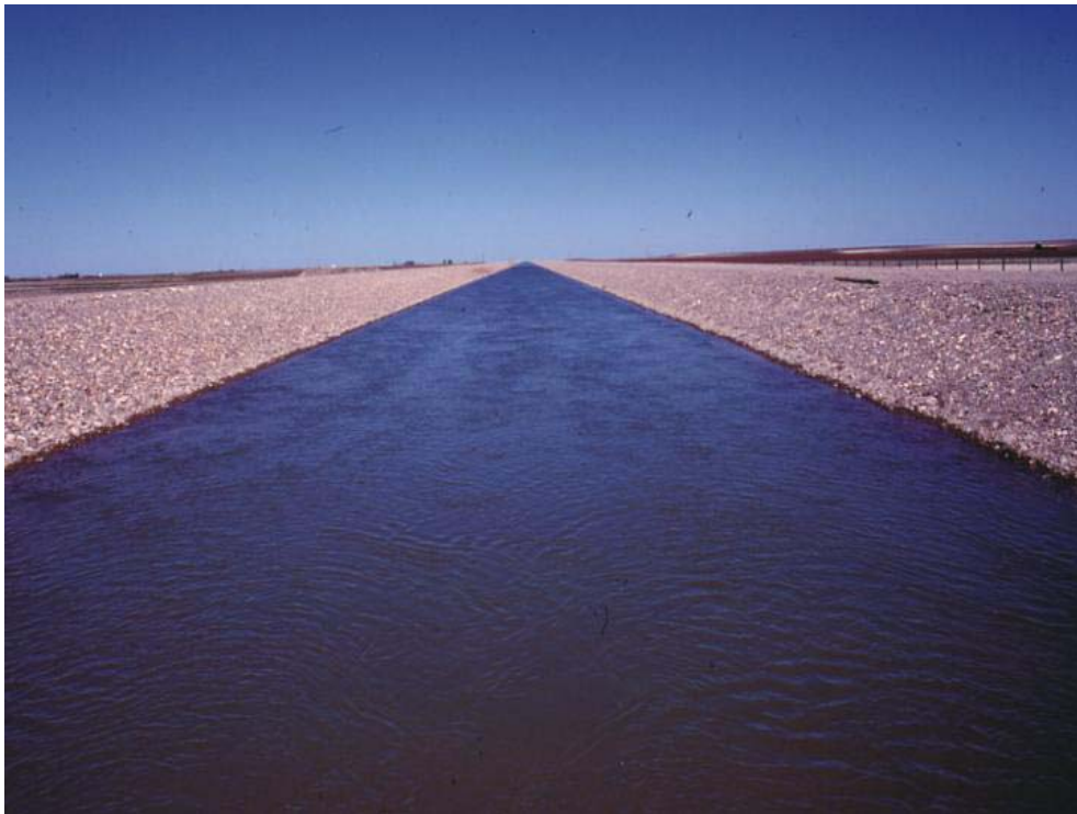
Lethbridge Northern Headworks Canal
