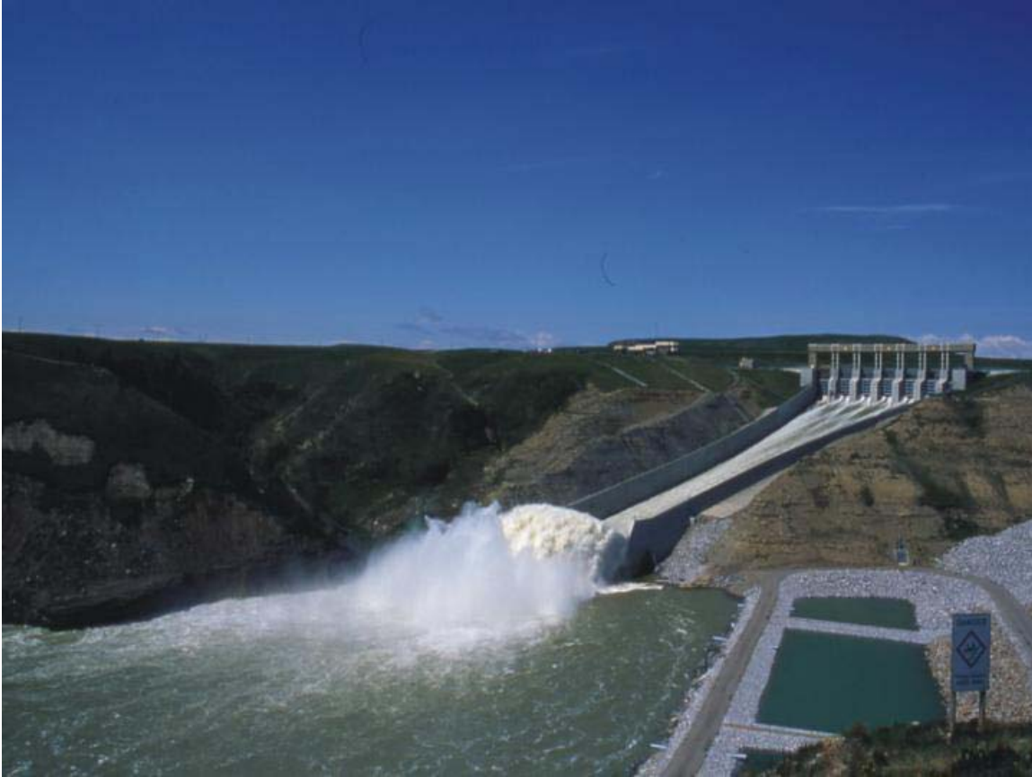
Oldman River Dam Spillway in Operation
