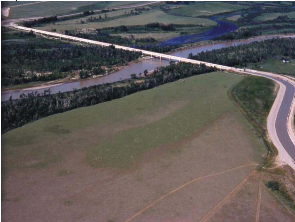
Lethbridge Northern Headworks - Oldman Flume and Canal
