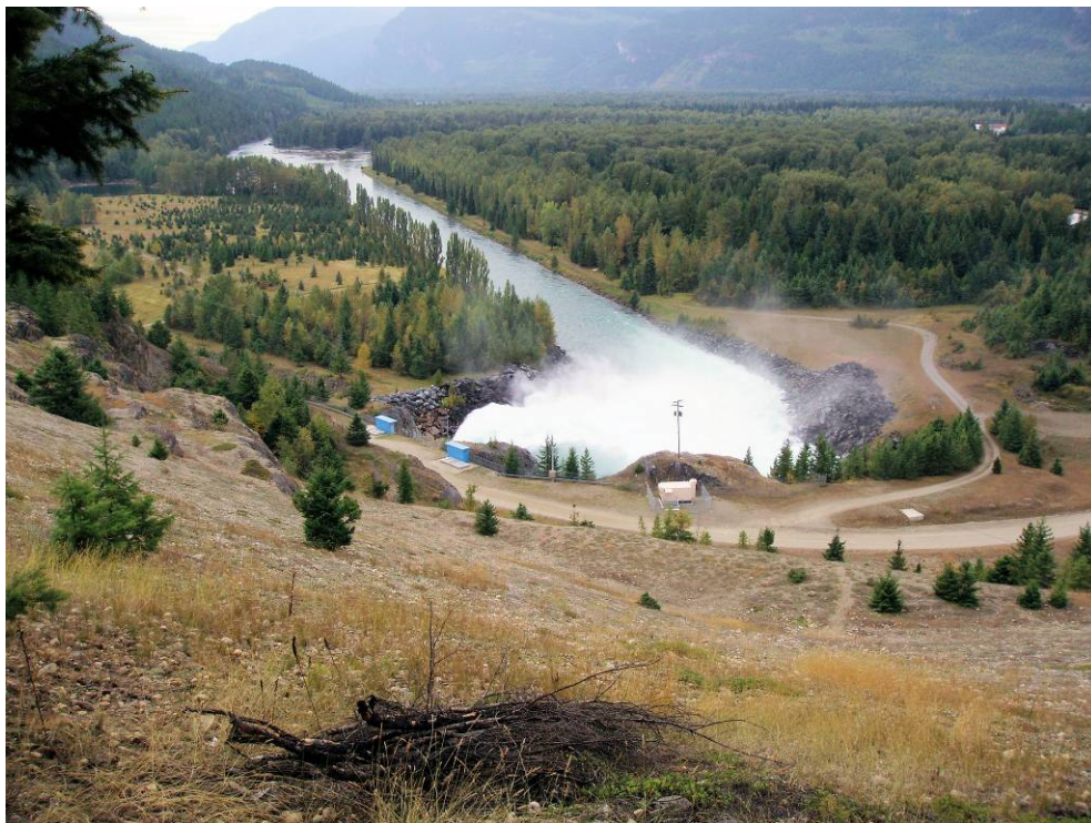
Number 1 tunnel in Duncan Dam releasing water at near-full throttle
