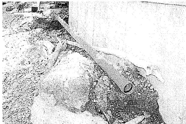
Broken Pipe 370.2/3nds Uncovered by removed March 2005
