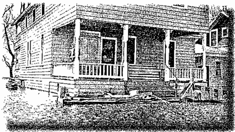
North porch of Huston cottage, 1952
